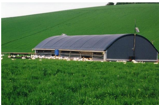
Figure 15 – Broiler arch with outdoor access
